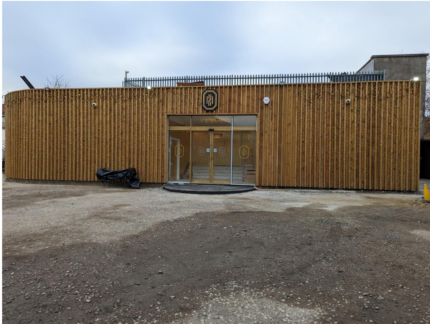
Photo 5 Rear facade and entrance (view from rear car park)
