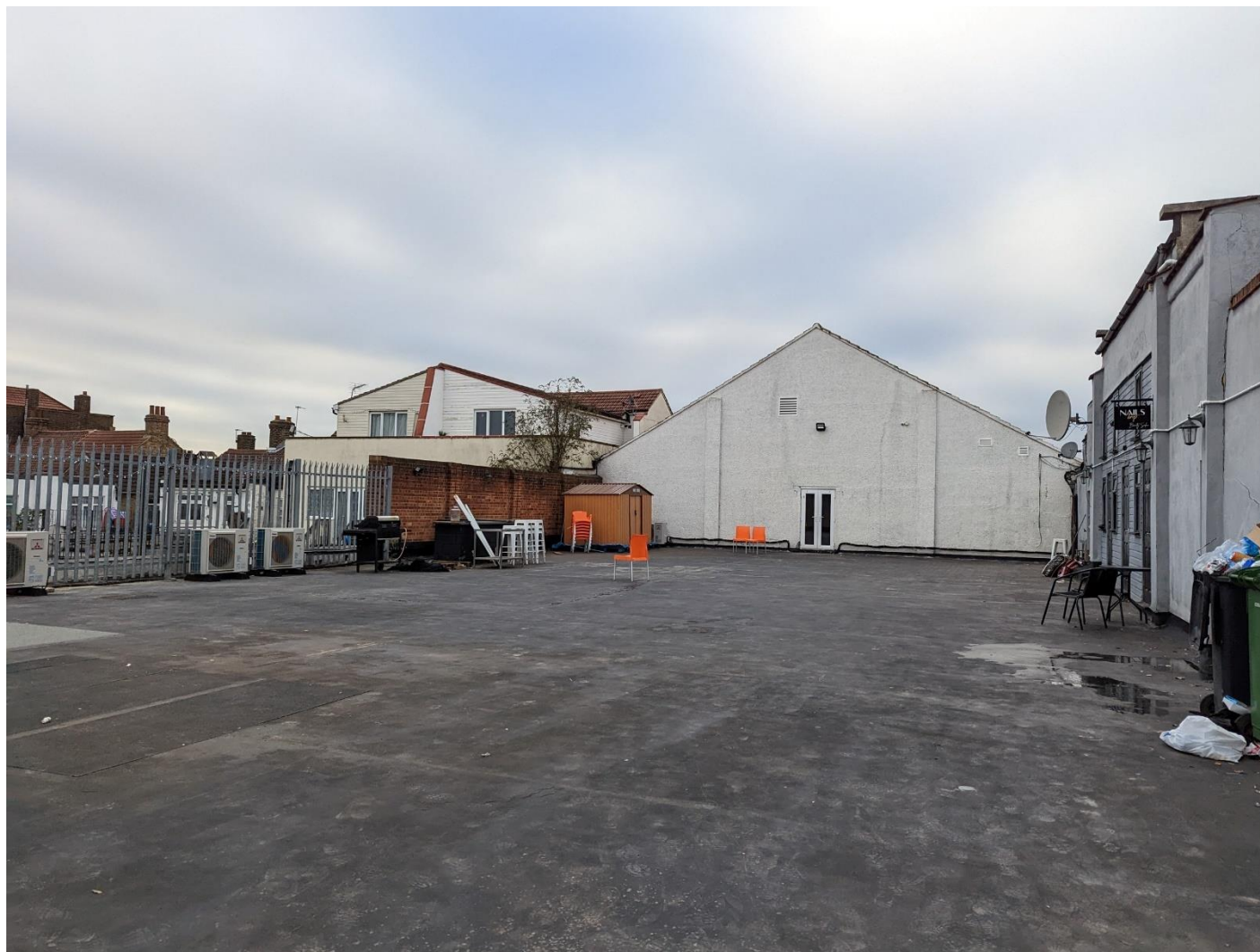
Photo 6 Flat roof (first floor level), facing west
